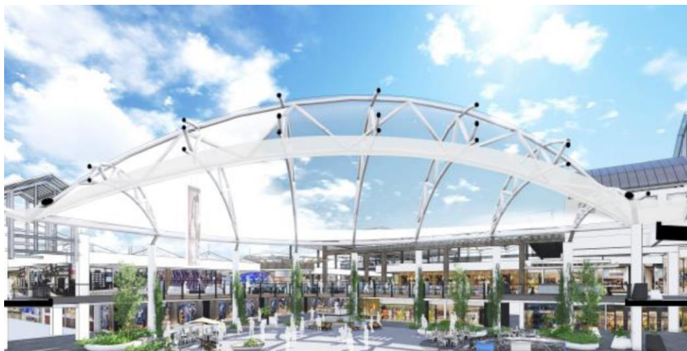
FIGURE 1 – CENTRE COURT OPEN AIR SHADE SAIL STRUCTURE (proposed as part of MOD2014/0230)
