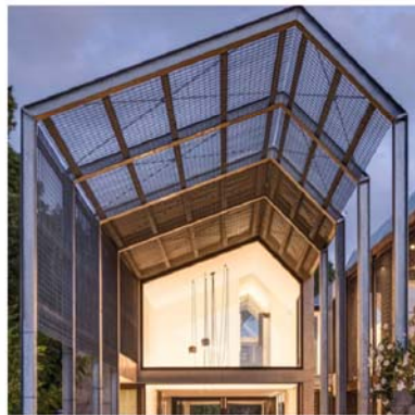
1 STEEL AND TIMBER FRAME STRUCTURE
