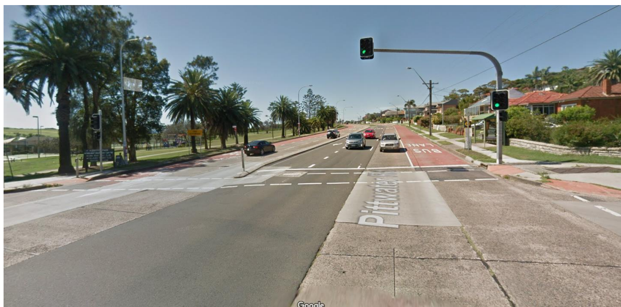
Figure 6 – Pittwater Road (facing south)
