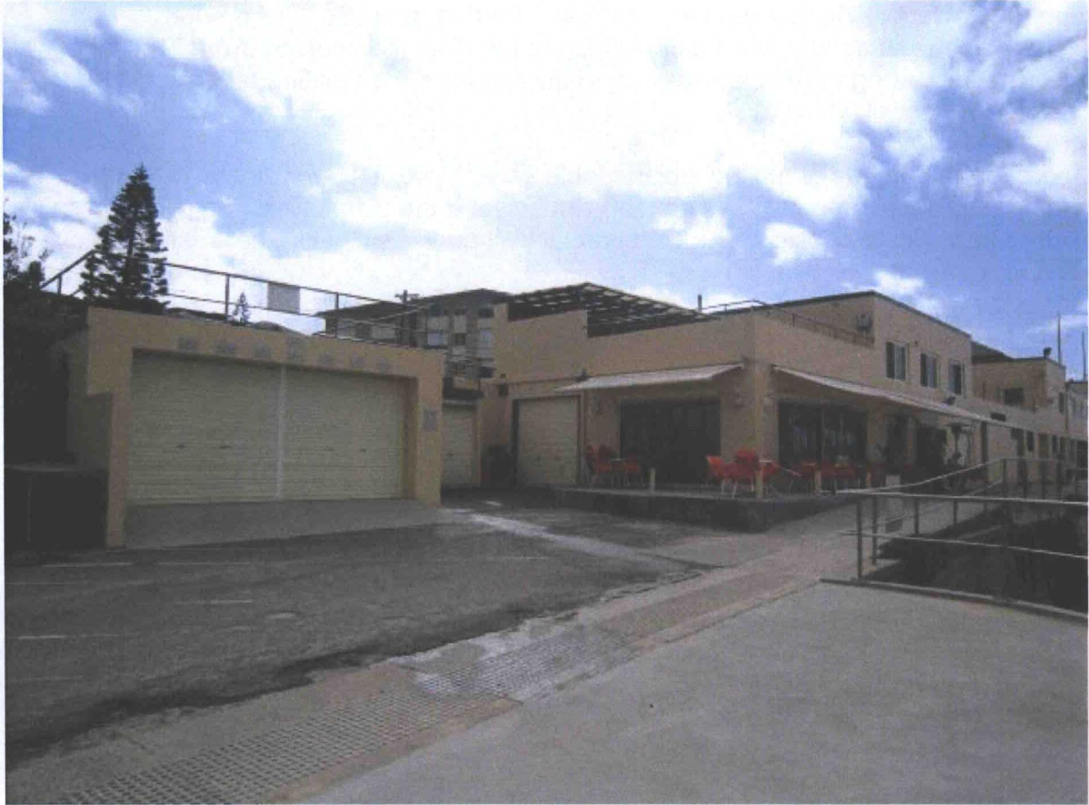
View of the southern end of the SLSC building from the ground level showing the area outside the café where the Grease Pit is to be located.
