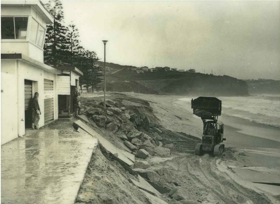
Figure 5: Rock revetment being placed seaward of Newport SLSC on 28 May 1974
