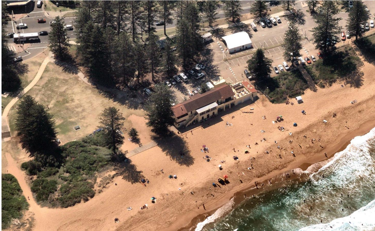
Figure 3: Oblique aerial view of Newport SLSC on 25 January 2021, facing NW
