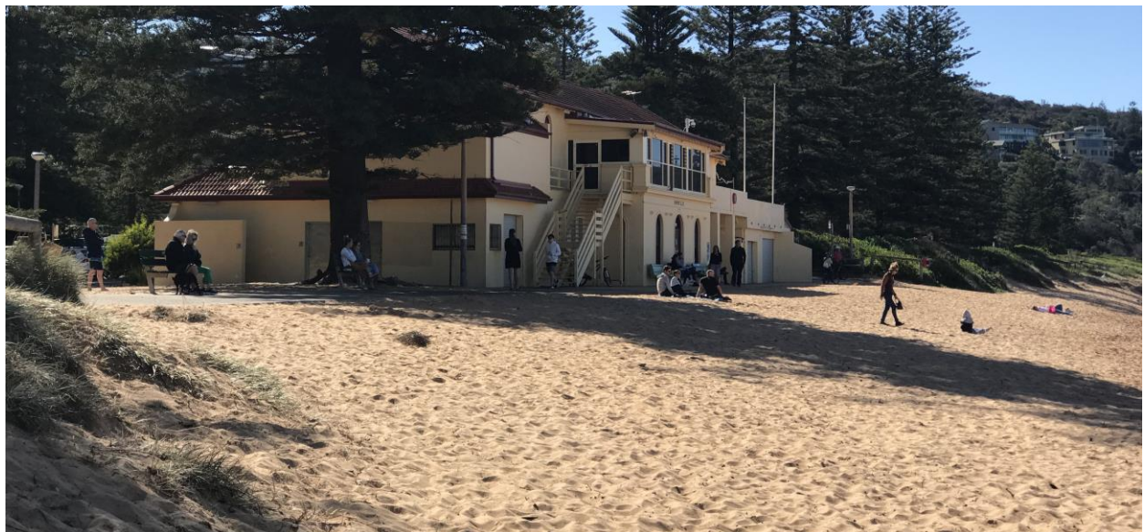
Figure 2: View of Newport SLSC building from Newport Beach on 17 August 2020, facing north
