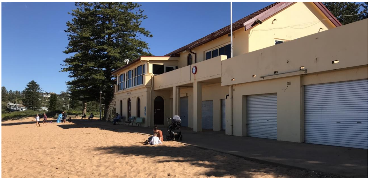
Figure 1: View of Newport SLSC building from Newport Beach on 17 August 2020, facing SSW
