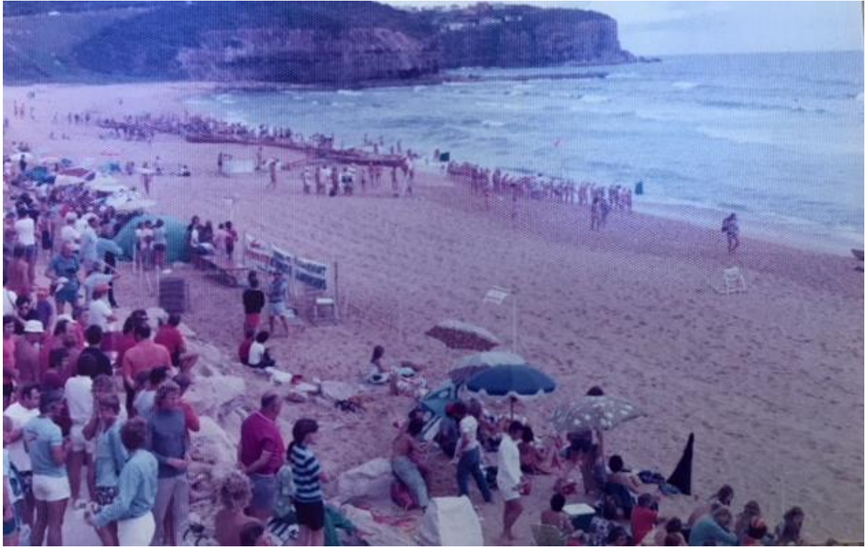
Figure 7: Rock revetment still visible seaward of Newport SLSC in February 1975
