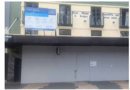
Reference Photo - Existing awning
