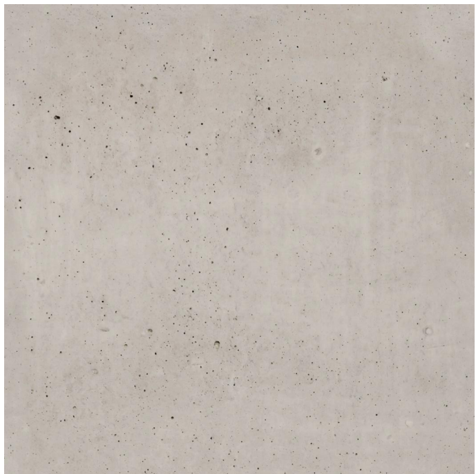
CONC NATURAL OFF-FORM CONCRETE
