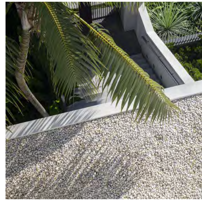
GR GRAVEL BALLASTED ROOF
