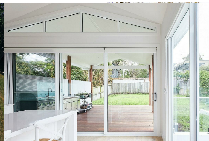
AL1 - Powdercoated aluminium windows and doors
