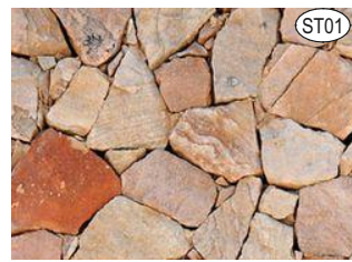
DRY PACK STONE WALL
