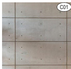
OFF FORM CONCRETE
