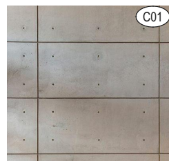
OFF FORM CONCRETE
