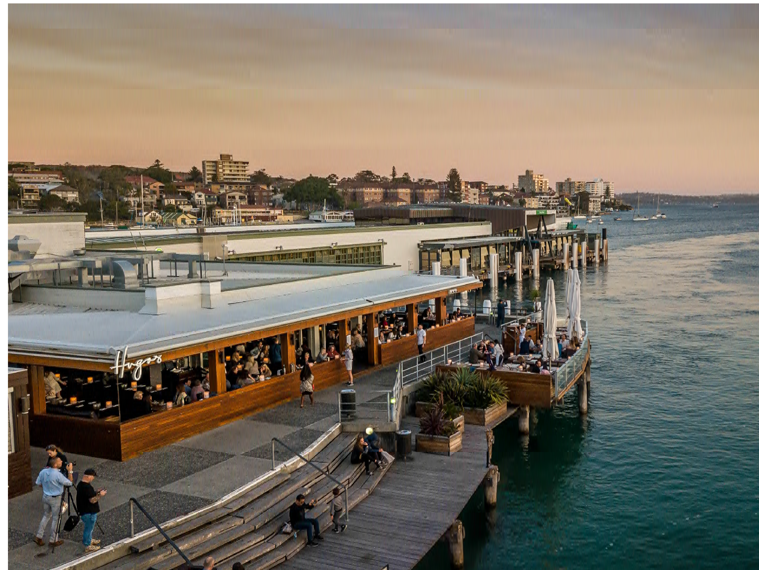
02 SITE PHOTO - DRONE PHOTOGRAPH OF EXISTING SITE AND CONDITION
