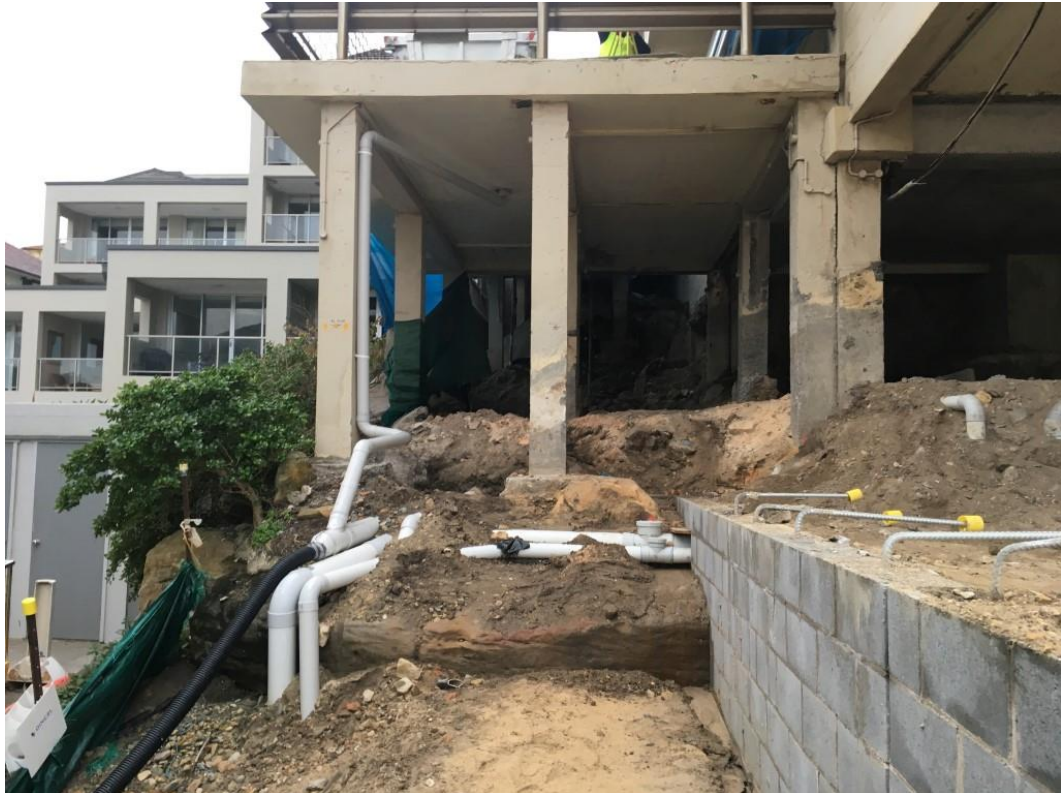
Figure 1 – Photograph showing depth of bedrock in the south eastern corner of the property with the block wall, now clad in stone as depicted in Figure 2, founded on bedrock along its length
