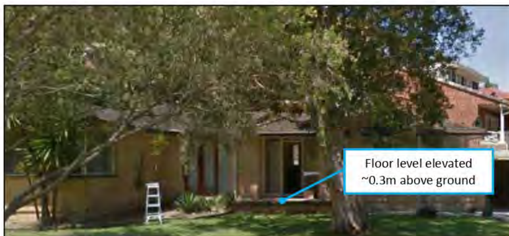
Plate 11 Example of a building on Howell Close with floor level roughly 0.3 metres above the surrounding ground surface
