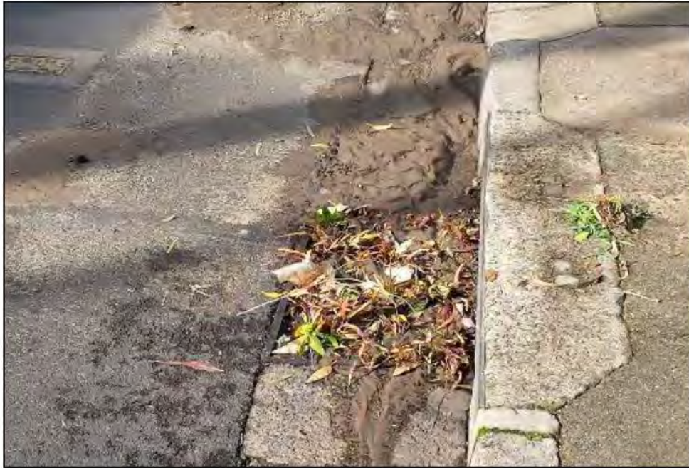
Plate 12 Typical blockage of a stormwater pit
