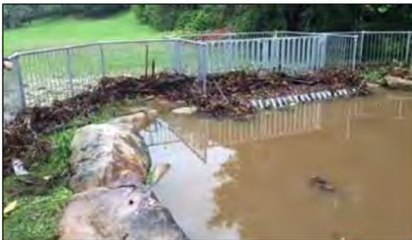
Plate 6 Flood levels and debris build-up at the Howell Close culvert inlet during the November 2015 flood
