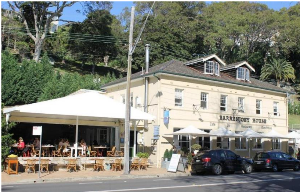
Figure 11: Barrenjoey House in 2015 prior to the most recent renovations.
