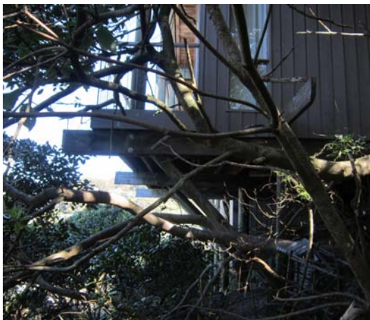
Site photo of the subfloor area and garden affected by the proposal
