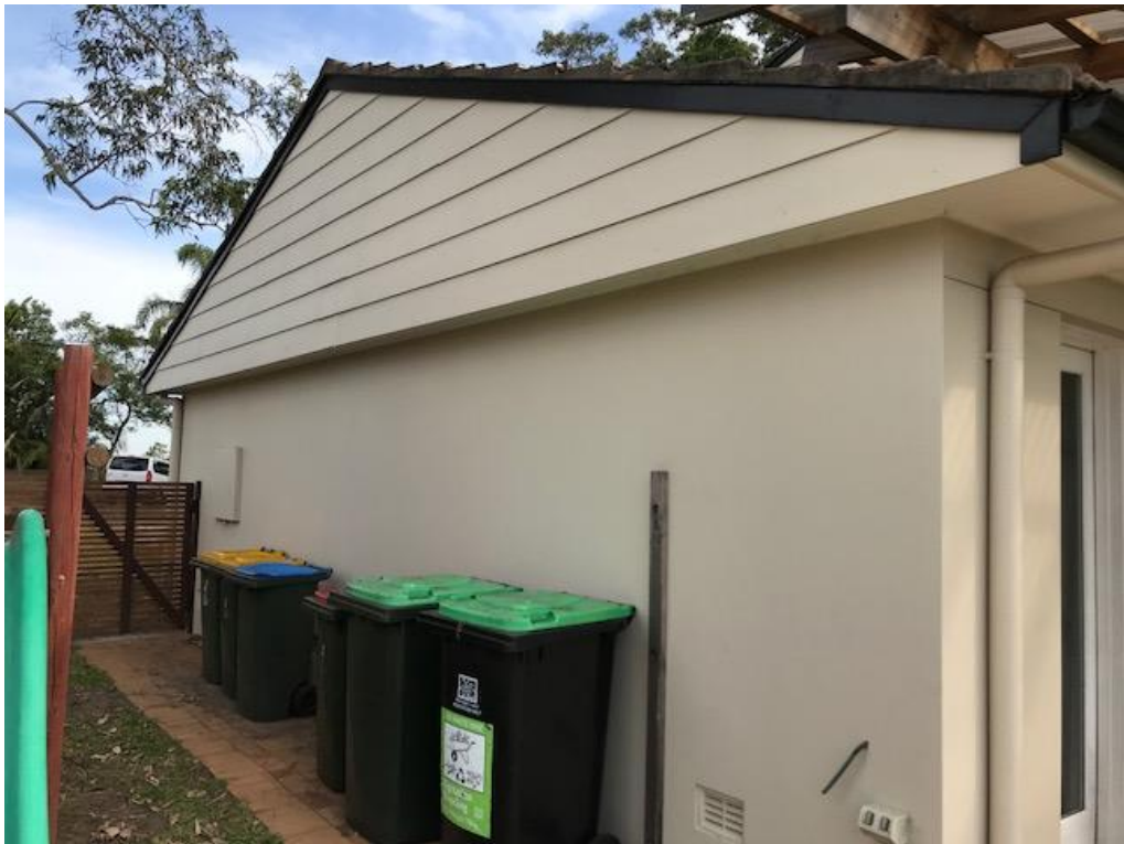
Figure 5. Existing garage and laundry
