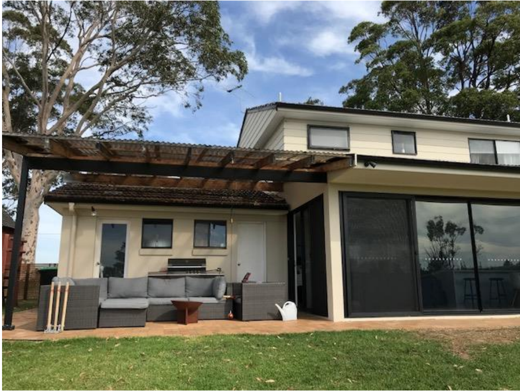
Figure 4 - The rear of the existing dwelling
