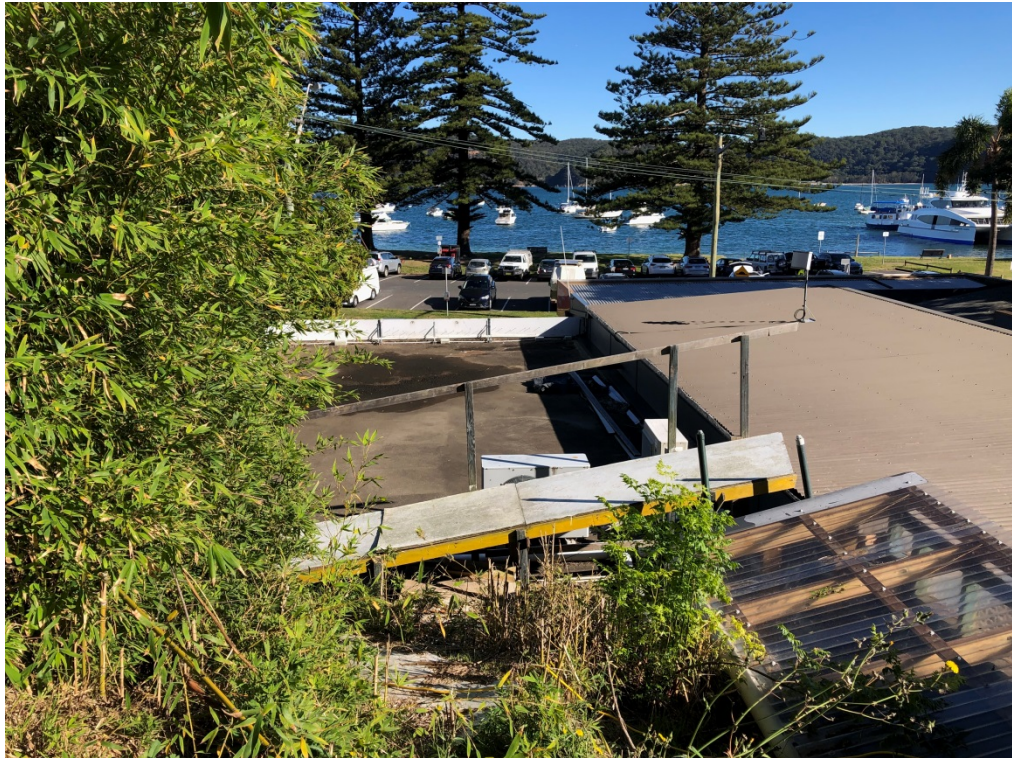
Photograph 9: View of roof of the shops, facing west (18/06/2021).
