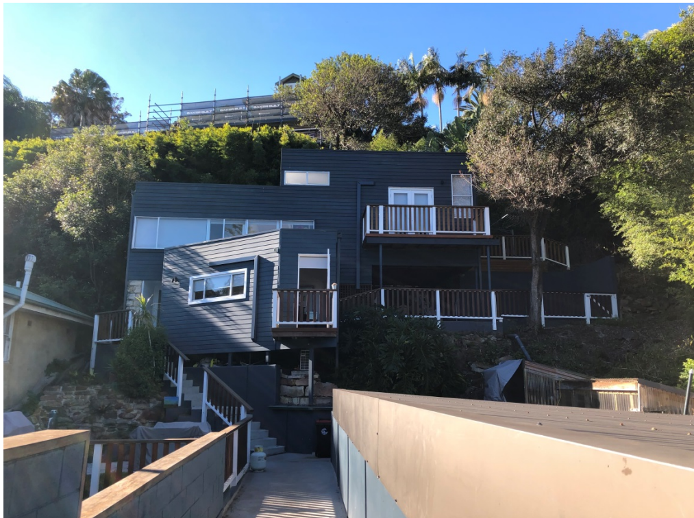
Photograph 4: Timber house on site, facing east (18/06/2021).
