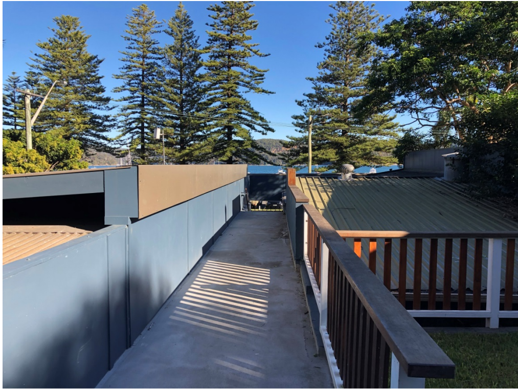
Photograph 3: Concrete stair and walkway, facing west (18/06/2021).
