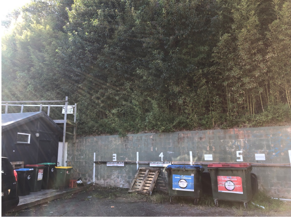
Photograph 5: Brick retaining wall at carpark area, facing northeast (18/06/2021).
