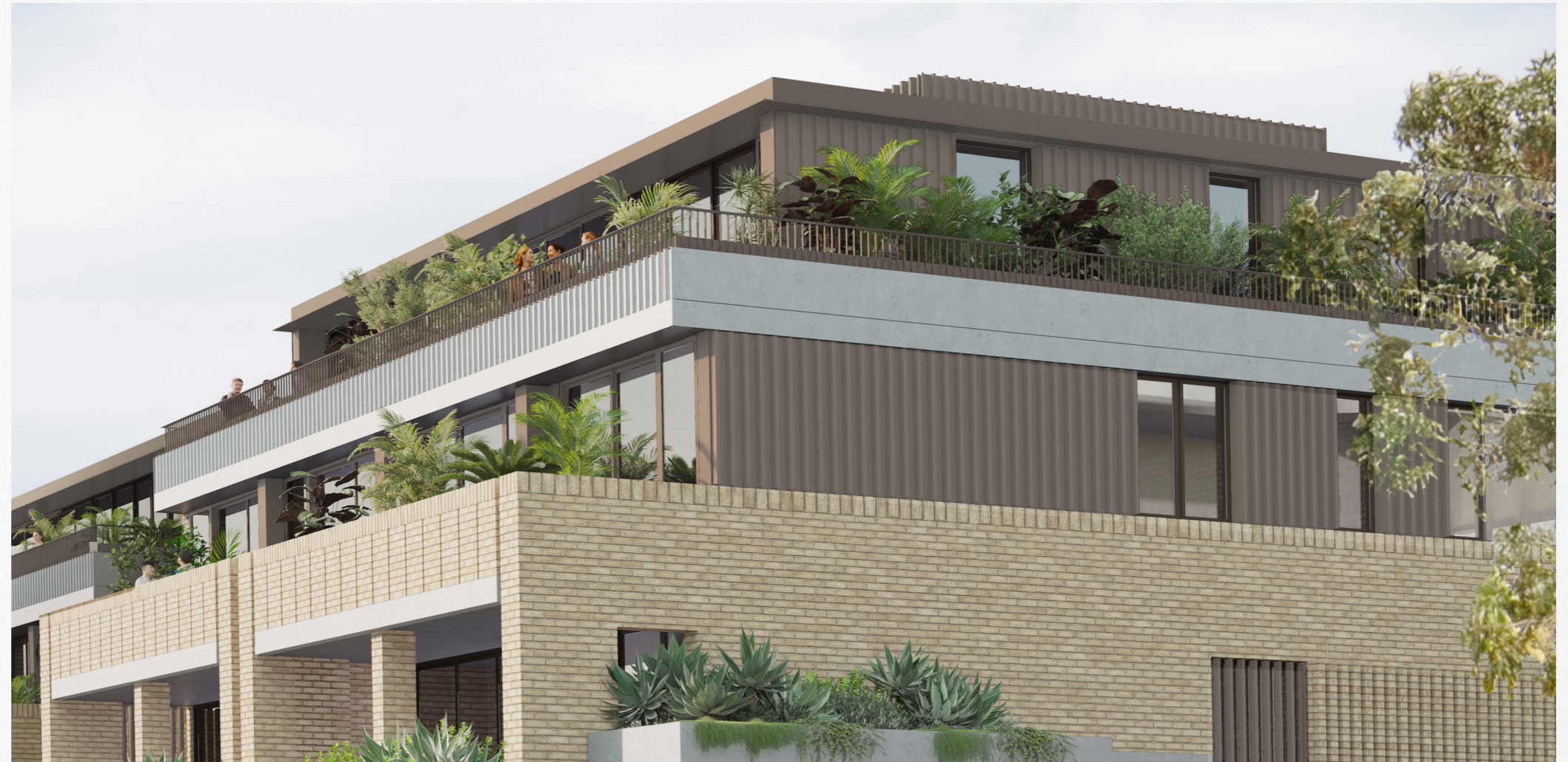
Artistic Impression: View looking towards the corner of Lawrence Street and Dowling Street
