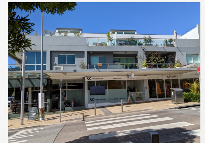
6 Site Photo - "The Caville" - 6-8 Lawrence Street
