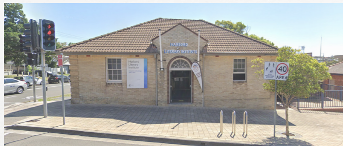
Site Photos: Materiality referencing local heritage items
