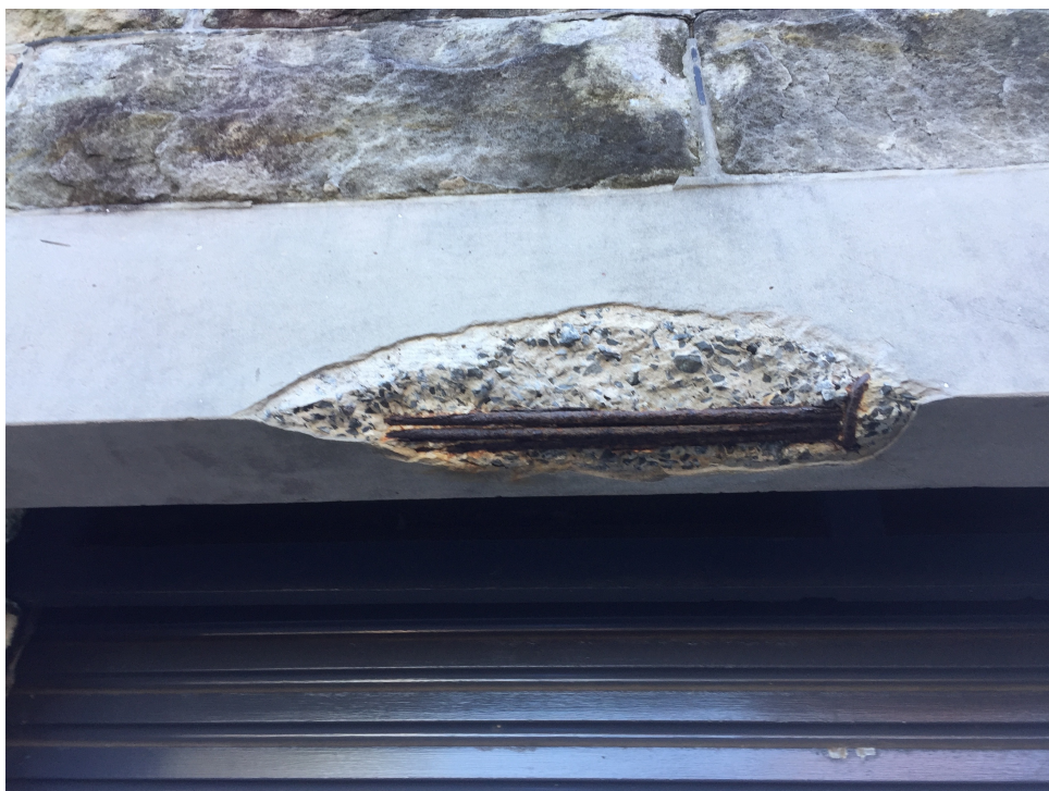
Photo 3: Concrete Cancer Source: apwdesign
