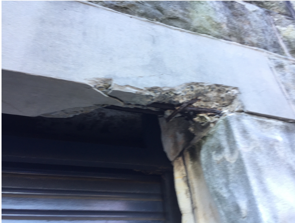
Photo 2: Concrete Cancer Source: apwdesign
