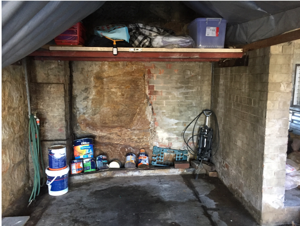
Photo 4: Dampness to garage Source: apwdesign
