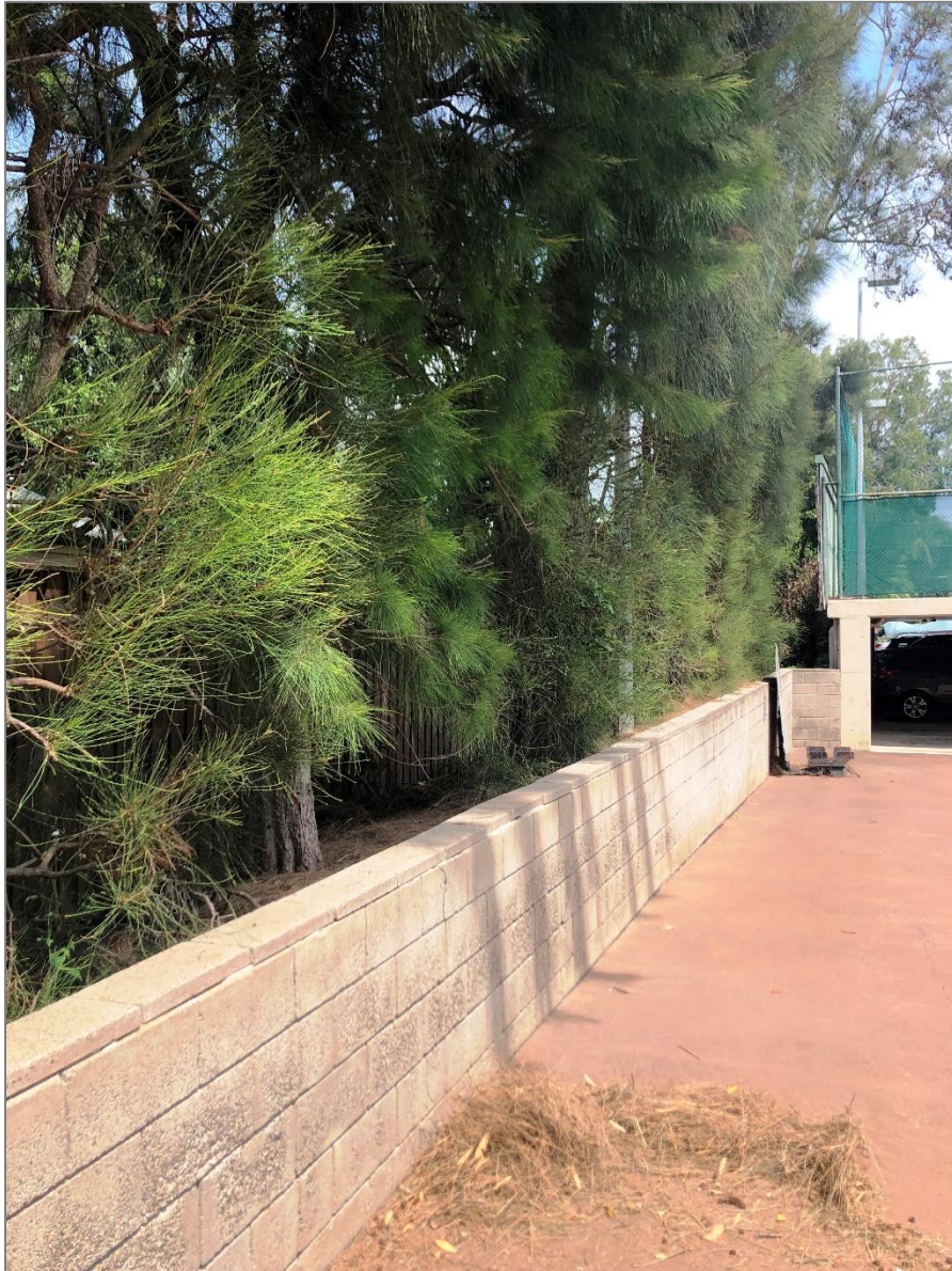
Plate 3 Group 13 – Swamp She-oak in raised garden bed, no sign of root ingress outside of retaining wall.
