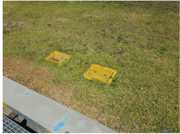
Reticulated water / hydrant in pathway
