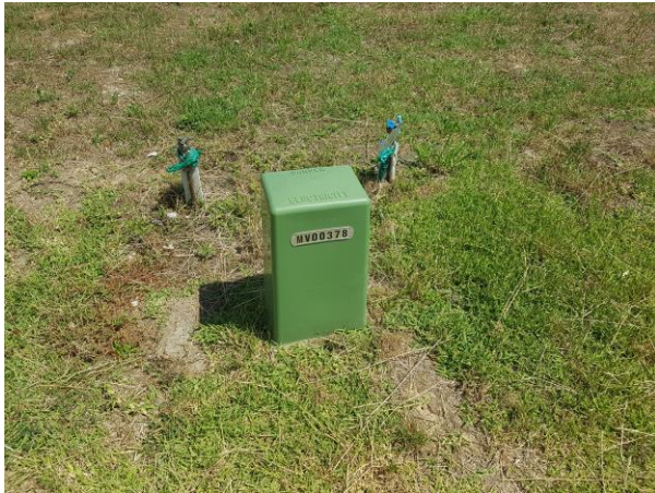
Existing underground electrical supply
