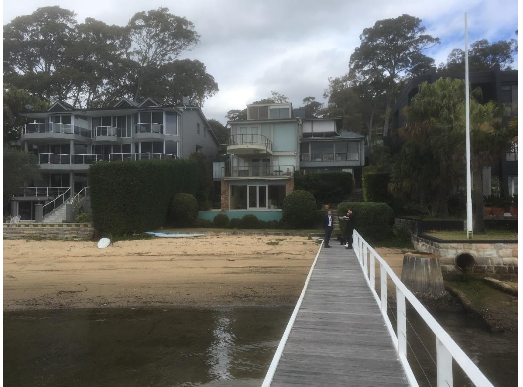
Figure 12. View of 1770 and 1772 from the foreshore. No impact due to breach of envelope as the rear facades harmoniously address the foreshore
