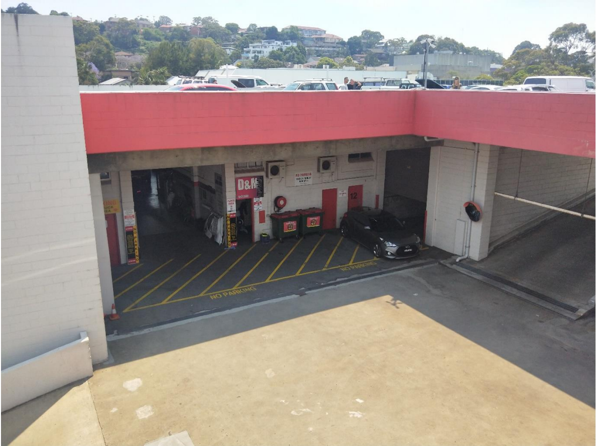
Figure 3: Oblique aerial view of Unit 12.
