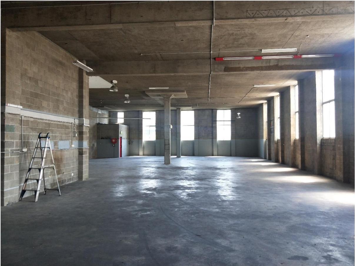
Figure 7: Photograph of the ground floor of Unit 12.
