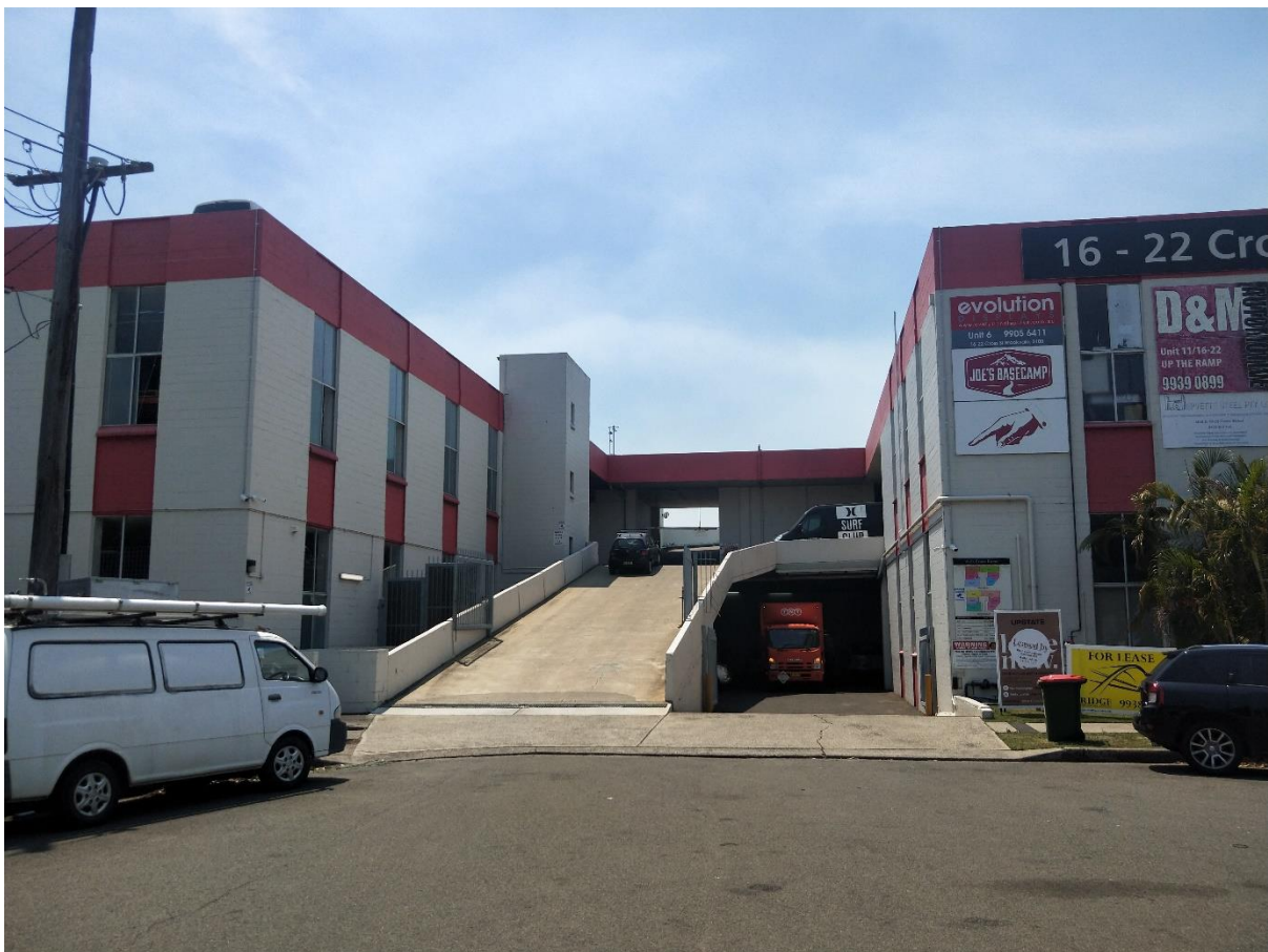
Figure 9: Photograph of the subject site when viewed from Cross Street.
