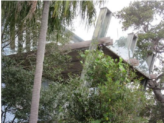
View to neighbouring residence outdoor area. Please note it is well elevated above the proposed work area.
