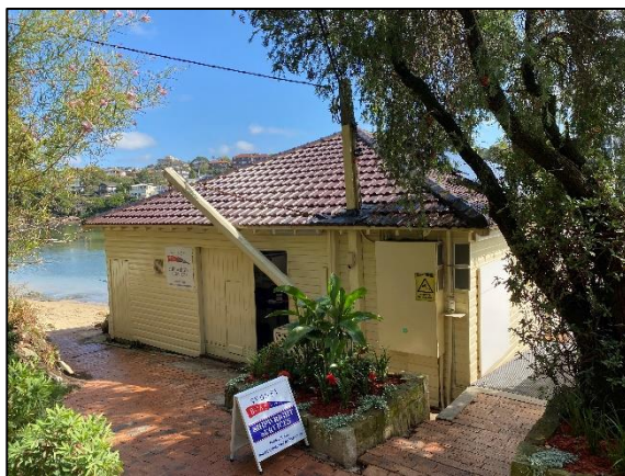
Photograph 1: The building, as viewed from Gourlay Avenue
