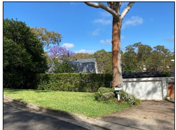
Photograph 11: No. 8 Gourlay Avenue, as viewed from Gourlay Avenue
