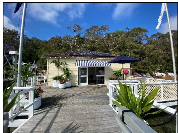
Photograph 2: The building, as viewed from the rear
