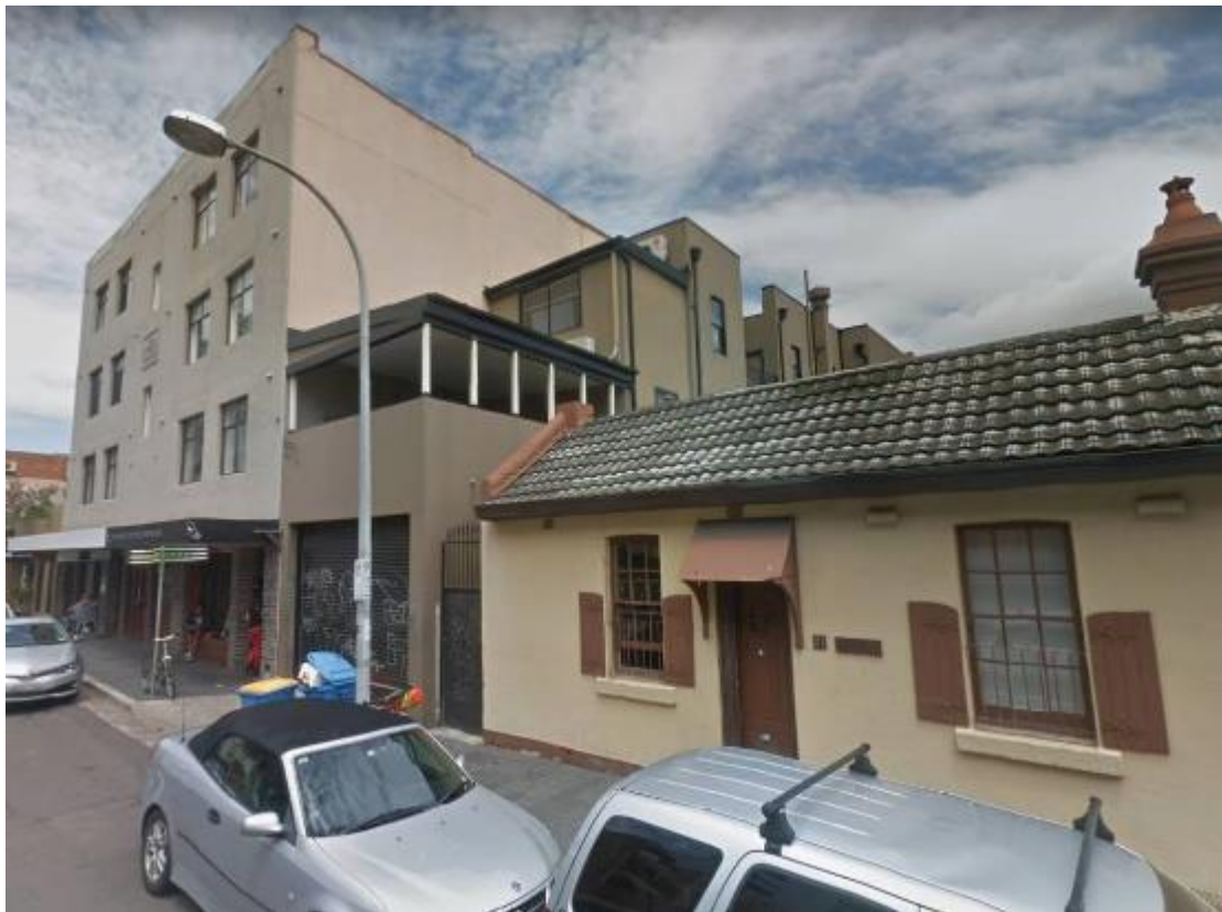
Figure 2 – Adjoining development to the south along Whistler Street
