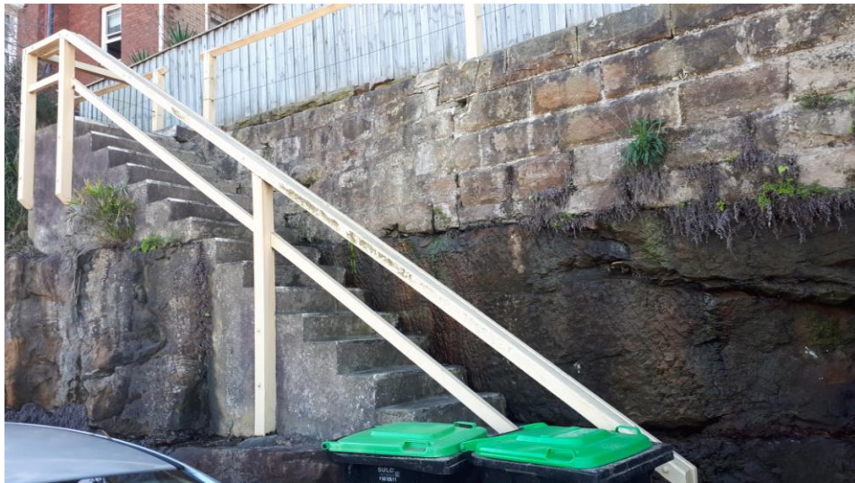
Photo 8: Existing stairway in front of property No. 58 Lauderdale Avenue
