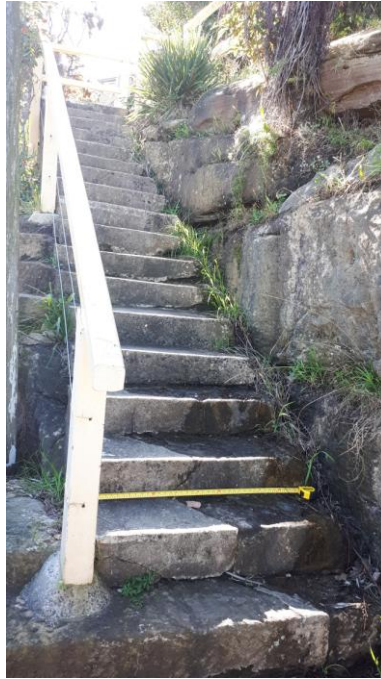
Photo 1: Existing concrete stairway leading from street level to upper foot path
