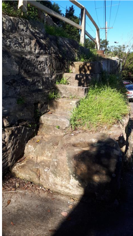
Photo 7: Alternative location for relocation of stairway
