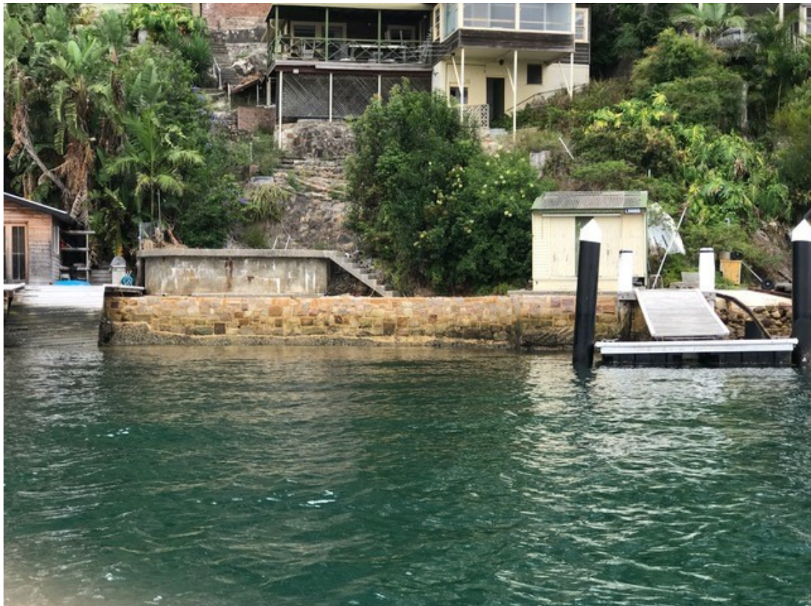
Photographs 1 and 2 show current degraded condition of existing shed
