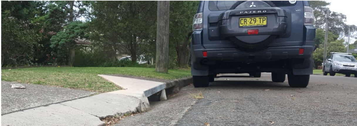
Figure 3. Existing on-grade pit (no grate) at 16/18 Dareen Street - side view with crest - photo looking downstream.
