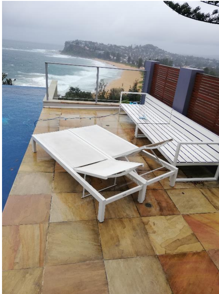
Image 7. View of Suspended Slab Adjacent to Pool Area
