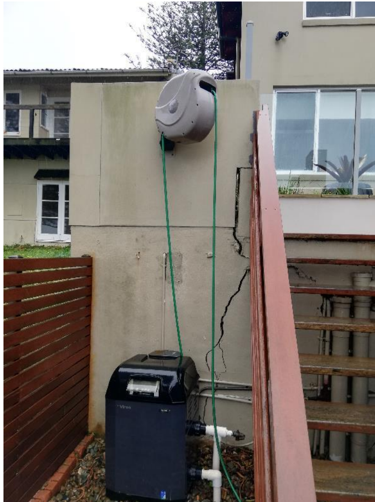
Image 1. View of Retaining Wall to be Replaced
