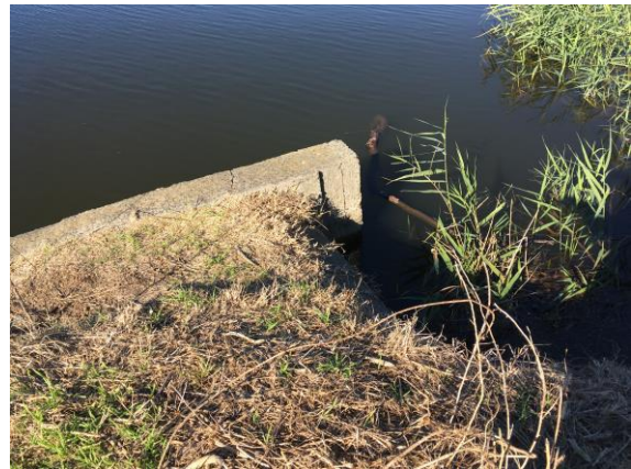
Figure 5: Erosion around edge of concrete headwall of stormwater outlet, looking south
