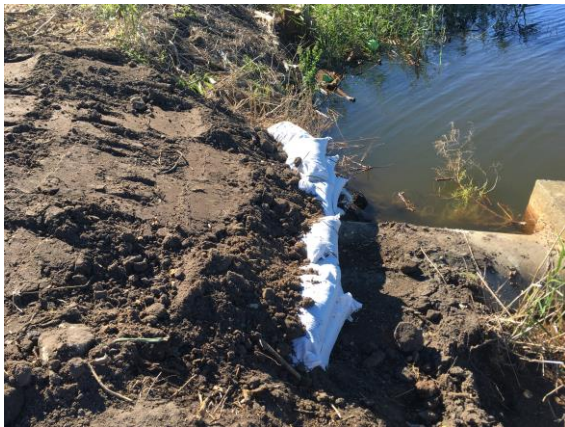
Figure 6: Sandbags behind recently repaired stormwater outlet, looking east
