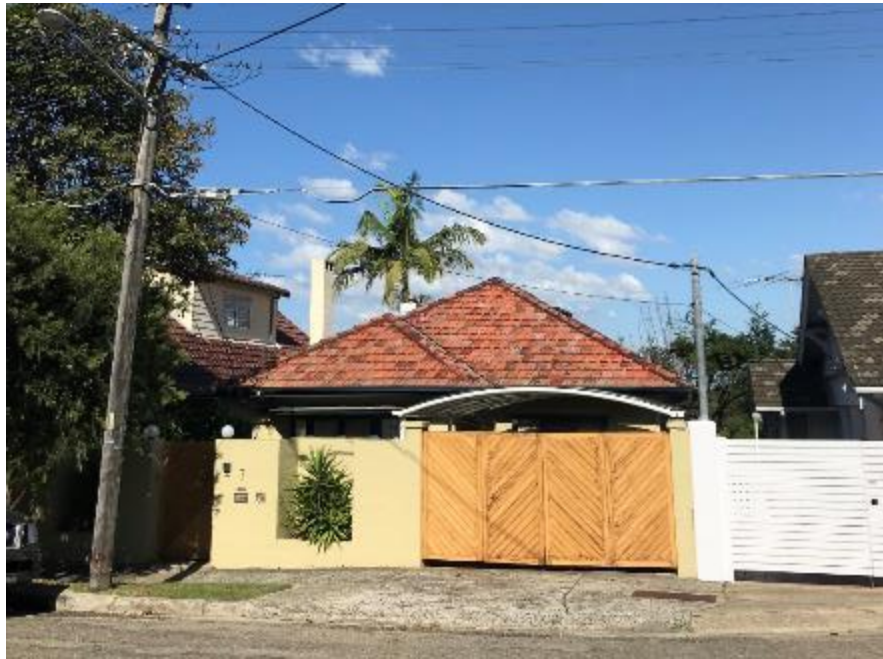
View of Subject Site from Street
