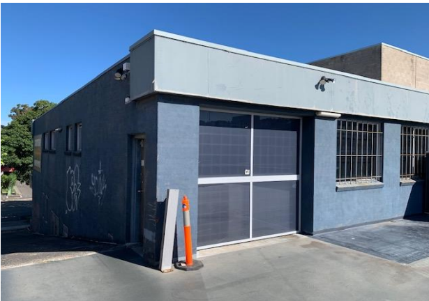
Figure 10: Existing full height retractable door
