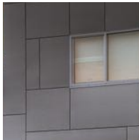
FC FIBRE CEMENT CLADDING NON-COMBUSTIBLE NOTE: COLOUR TO MATCH EXISTING DWELLING DULUX: MALAY GREY
