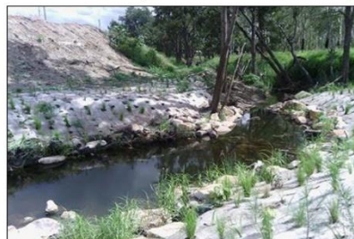
Plate 4 – Bundamba Creek Restoration works (Australian Wetland Consulting, 2018)
