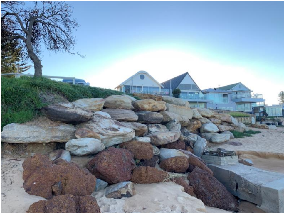
Photograph 4: Adjacent coastal protection works upgrades at Ramsay Street. Note these works were implemented by Council following the 2016 East Coast storm event and were not subject to DA approval
