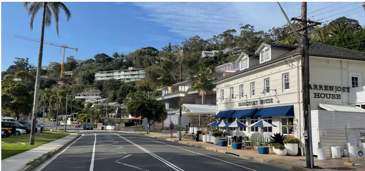
Figure 11- Photomontage showing the proposed development relative to its established built form context, including Barrenjoey House, as viewed from Barrenjoey Road.
