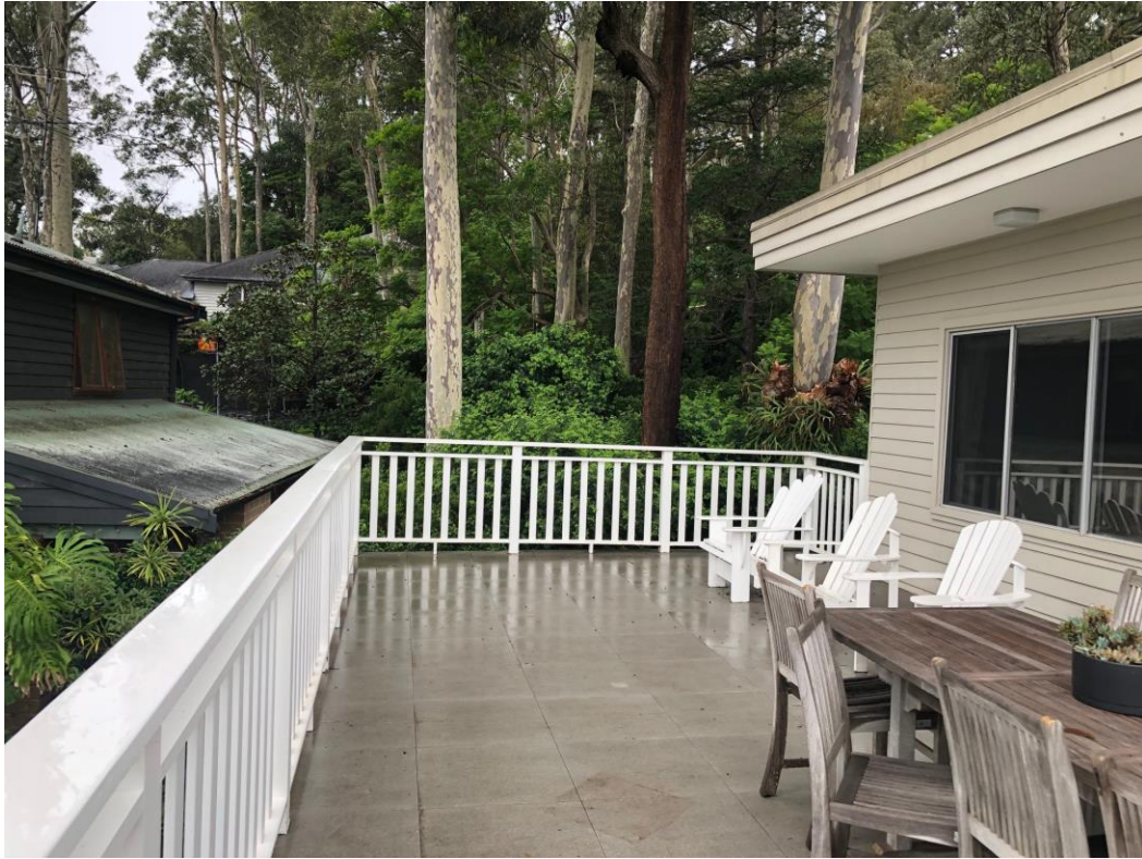
Figure 6 Existing deck and location of new proposed roof looking east
