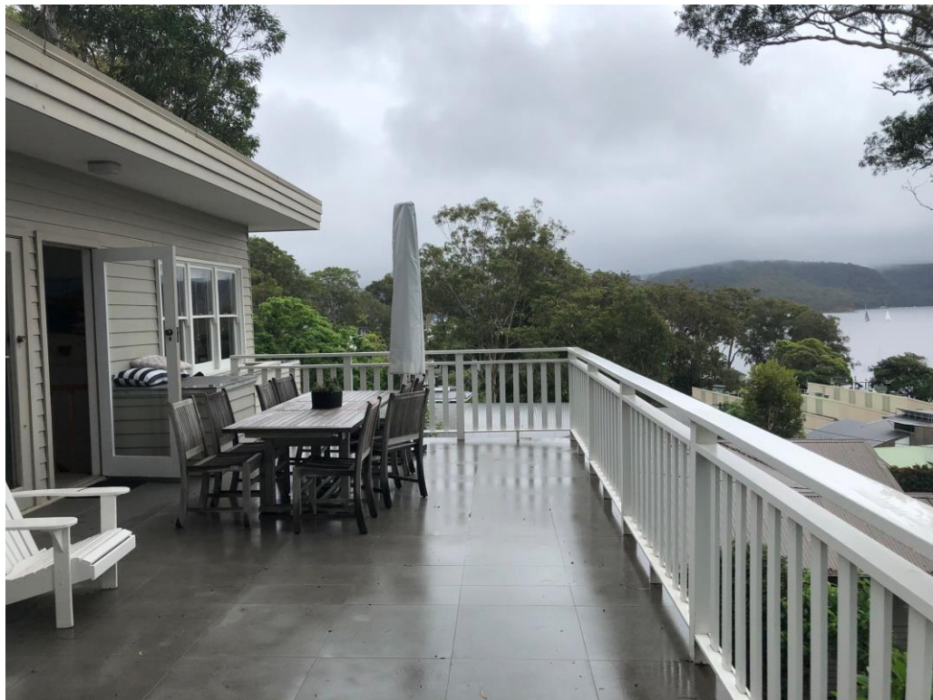
Figure 5 Existing deck and location of new proposed roof looking west
