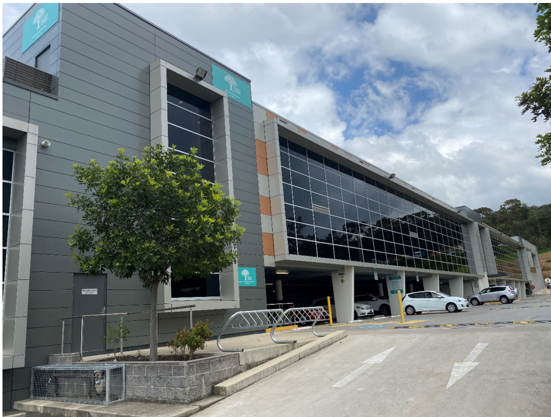
Figure 2 – Photograph of exterior of building.
