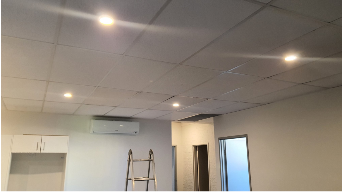
Photograph No. 1: Acoustic SMF containing ceiling tiles in Unit 3
