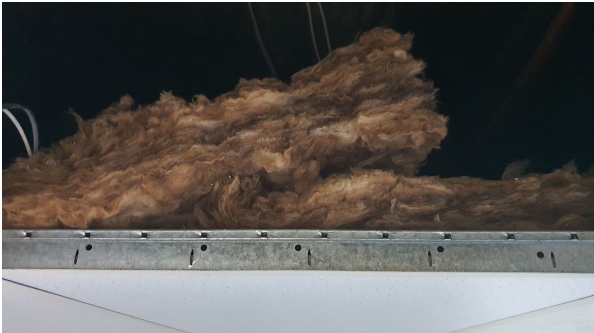
Photograph No. 2: SMF insulation batts on upper surface of ceiling tiles in metal grid ceiling
