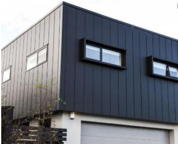
Denotes James Hardie Scyon Axon Cladding (Typical). Builder To Confirm Type & Colour
