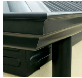
SETTLERS GUTTER PROFILE. 'BASALT' OR SIMILAR TO MATCH EX'G GUTTER.
