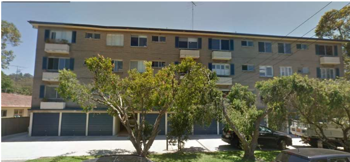
Figure 8: Photograph of the residential flat building at 12 Gladstone Street
