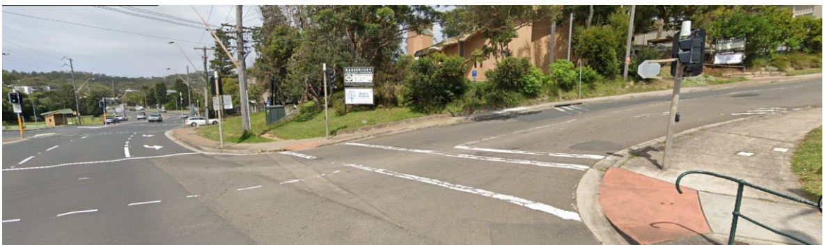
Kevin Avenue footpath and kerb ramps at Barrenjoey Road
