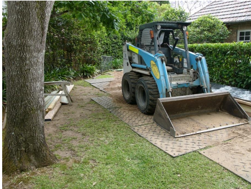
Figure 4 – Showing typical detail for truck mats.
