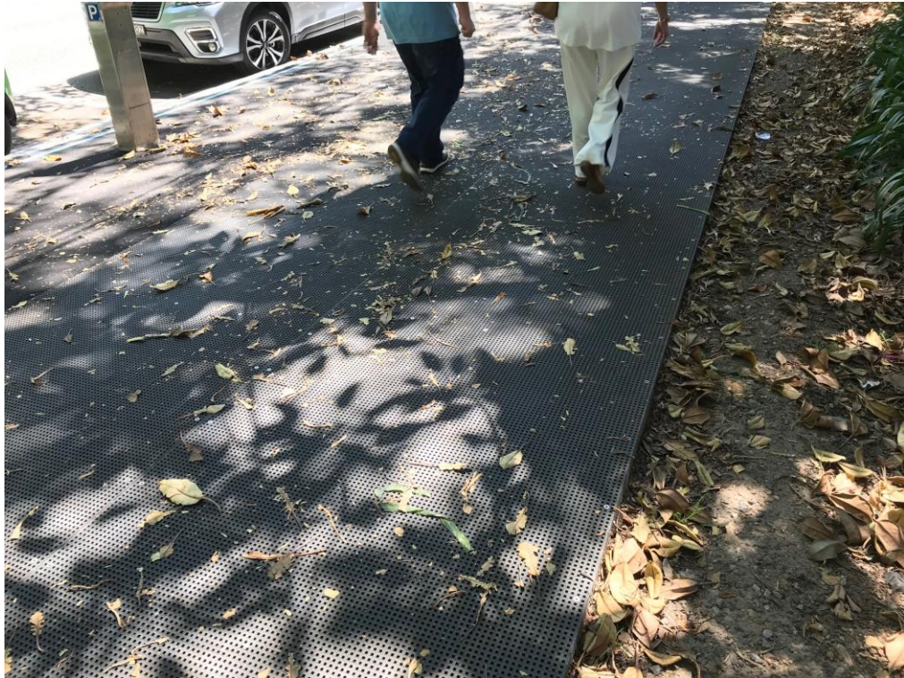
Plate 1 – Typical elevated FRP walkway (St. Leonards Park, North Sydney)
