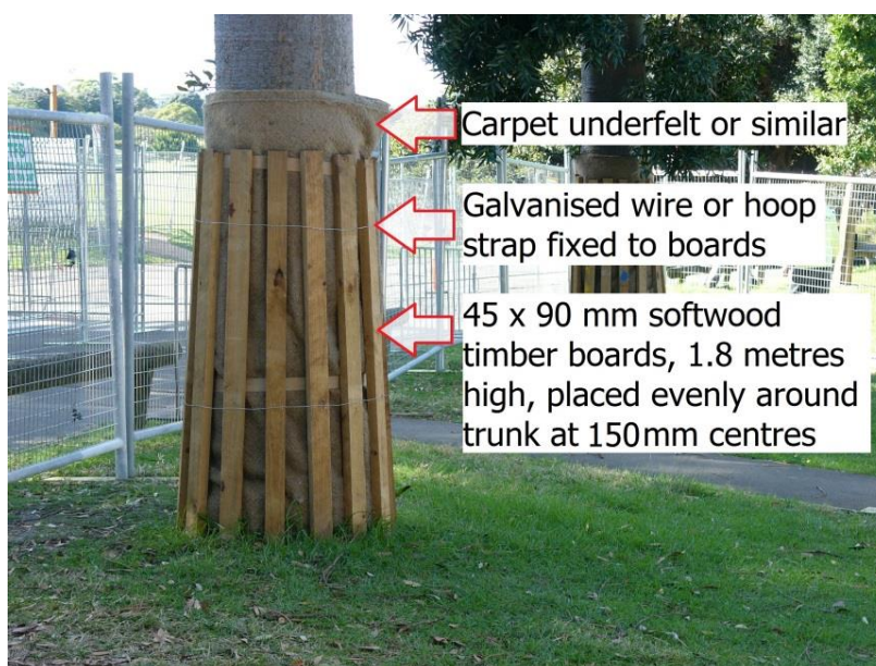
Figure 3 – Detail of Trunk Protection
