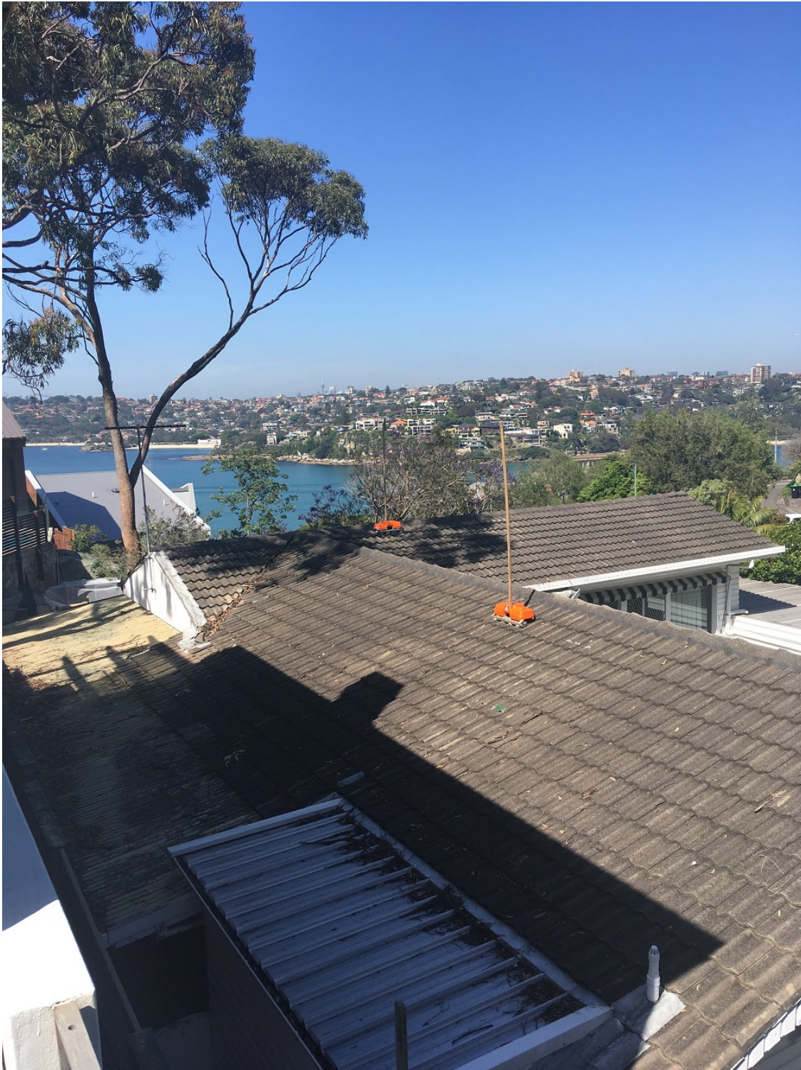
Photo 3. View from No. 57 Cutler Road side/front deck.
