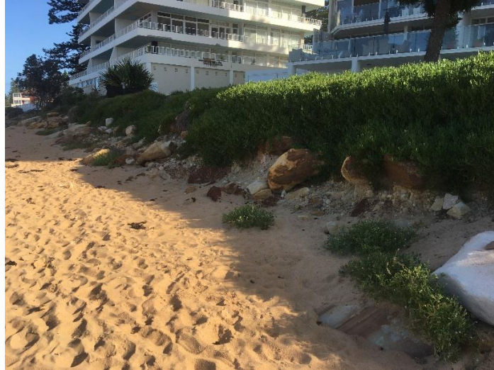
Photo: 1 – View of site showing informal boulder stabilising at rear of lawn.
