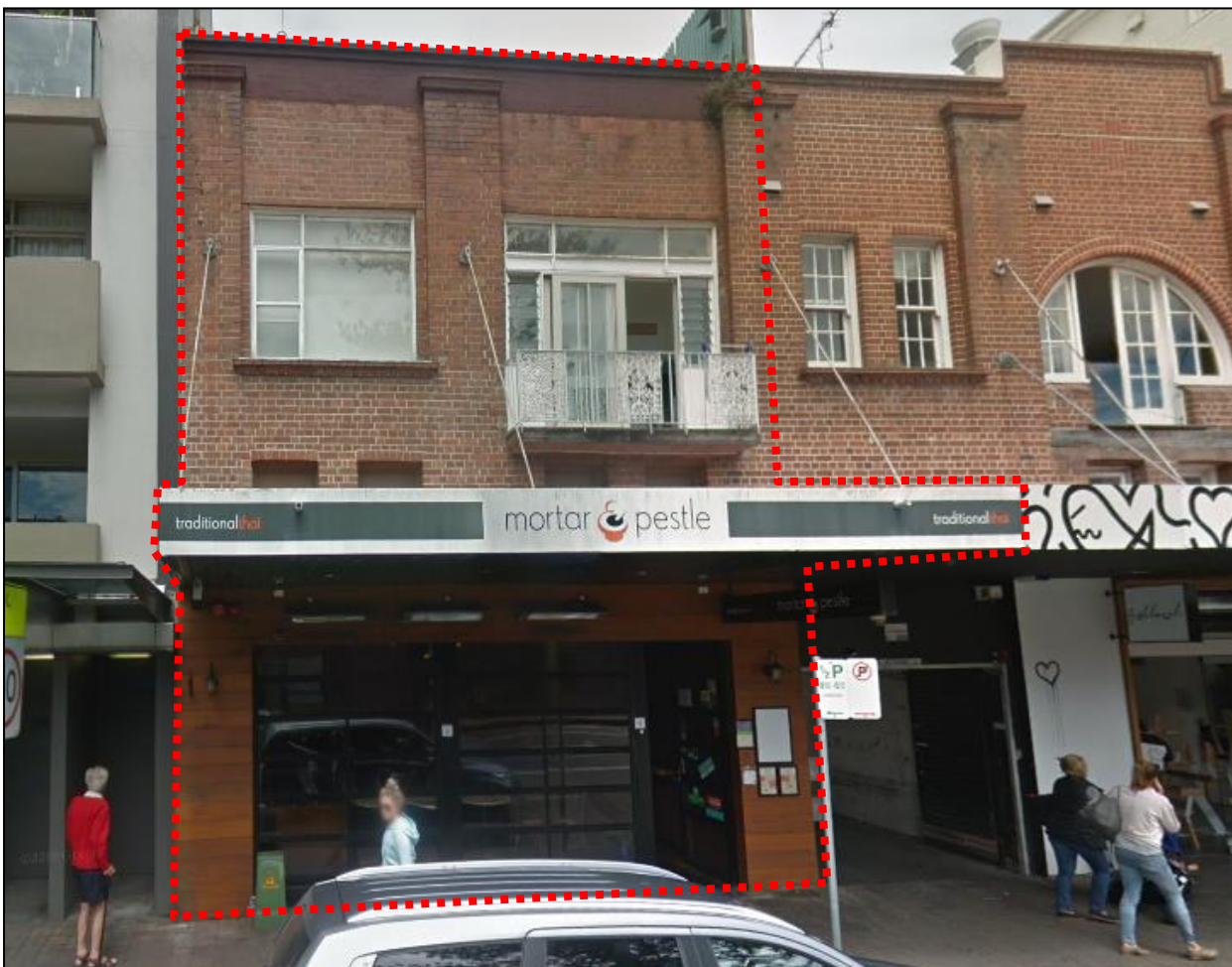
Figure 03: Neighbouring property at No. 2 Darley Road (Google Maps, accessed 2020)
