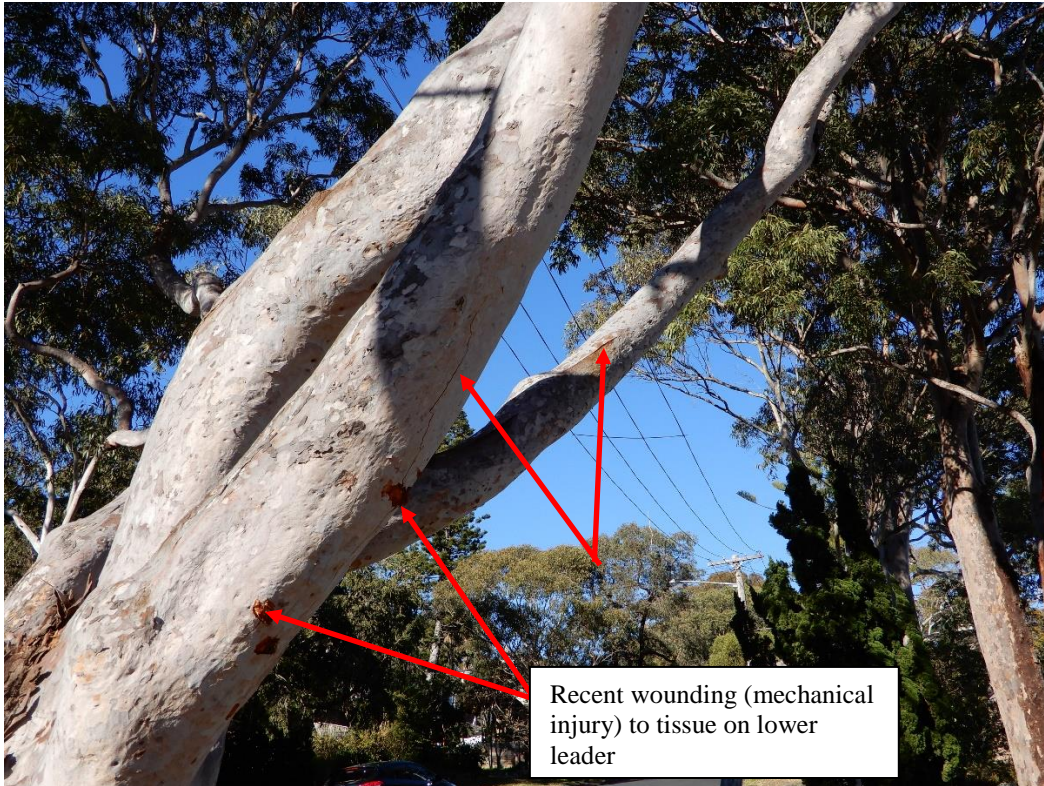
Photograph 7: Tree # 3 – Illustrating minor cracking in 2 lower leaders on west side.
