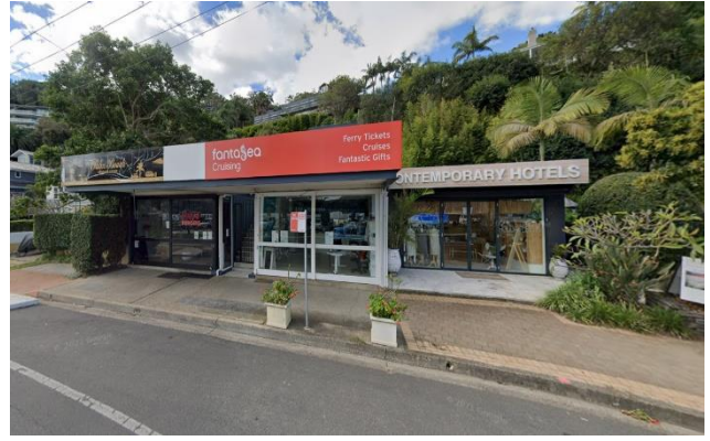
Figure 18 - Existing commercial buildings on site, now vacated.
