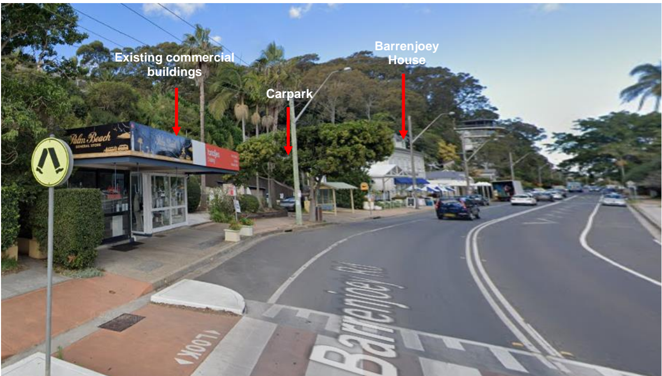
Figure 16 - View of subject site from Barrenjoey Road with Barrenjoey house indicated.
